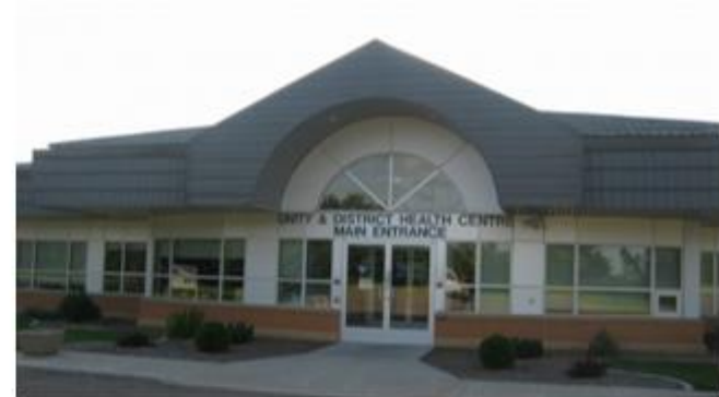
Unity & District Health Centre
