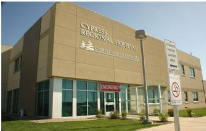
Cypress Regional Hospital – Swift Current
