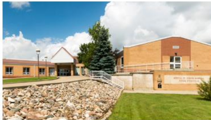
St. Joseph's Hospital – Gravelbourg
